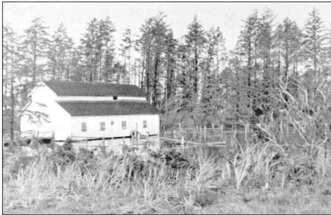
SUBMITTED BY SHANNON SMITH Shannon Smith's livery as it stood in the 1930s. Smith has been trying for several years to renovate the facility and use it for an events center.
