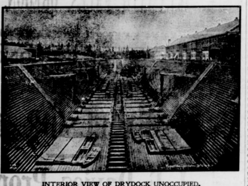
INTERIOR VIEW OF DRYDOCK UNOCCUPIED.
