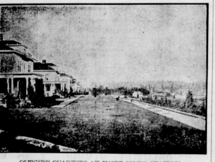
OFFICERS' QUARTERS AT PUGET SOUND STATION.
