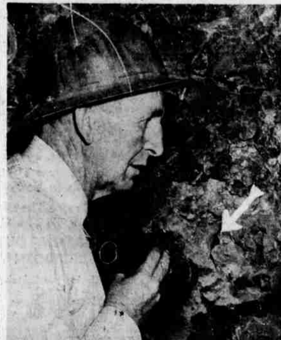
Willard Smith, associate reclamation engineer in charge of the tunnel project, looks with his flashlight into the drilled hole after the bit and rod are removed. Arrow points to the end of the hole. Explosive was later tamped into the hole and the wall blown out to open the 6600-foot of tunnel through the mountain.
