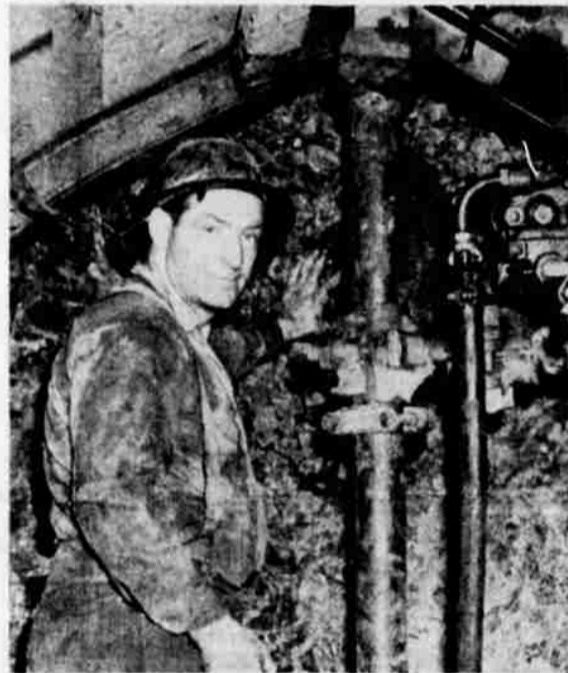
The tap-tapping of the west side drill can now be heard through the rock, and R. L. Welborn, shift boss, feels the wall for vibrations which may indicate where the drill will break through.
