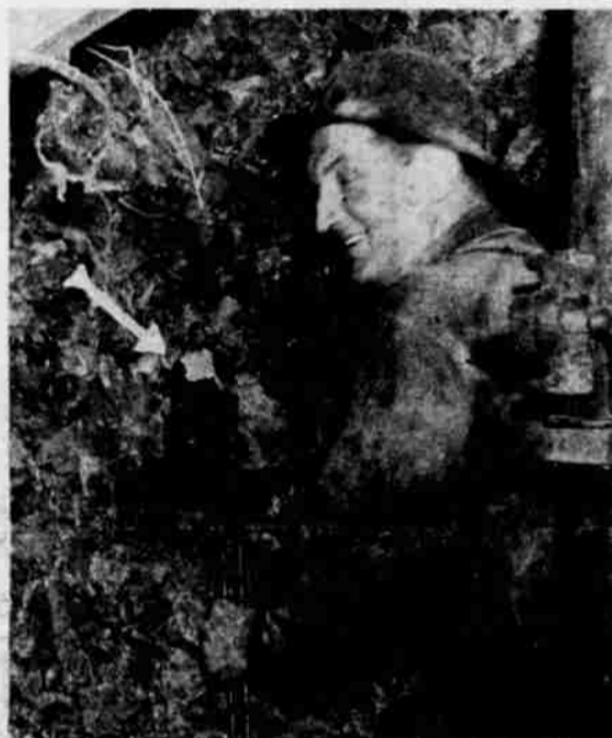
There she comes. Arrow points to the bit that cut the last wall. It is on the end of a nine-foot steel rod attached to an air-compressor drill on the other end. Welborn hooked the wrench around the rod to prevent the west side driller from drawing it back into the hole before the picture could be taken.
