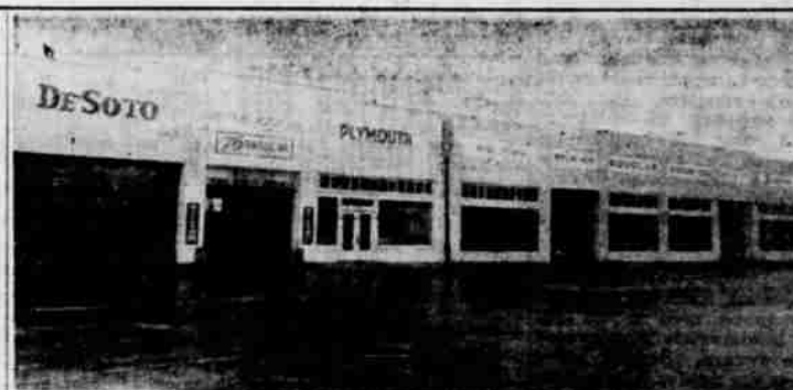
744-734-724 ENTIRE DOUGLAS MOTOR COMPANY SERVICE AND NEW CAR SALES DEPARTMENT
