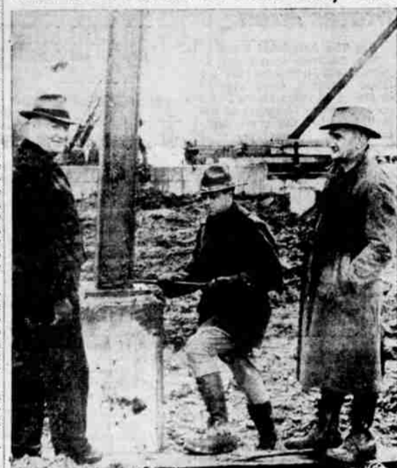
Construction of the Army's new huge $3,500,000 Utah general depot project northwest of Ogden rolled into high gear with bolting of the first steel into place by Captain Ruon J. Ballard, center, as construction officials watch. The warehouses will be used for storage of Army supplies for use of units west of the Mississippi.
