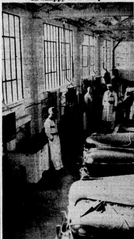
This picture was taken in the bright, shiny interior of the shop of the Marshall Cornett company. Oldsmobile dealers, who will occupy the new building at Seventh street and Klamath avenue Saturday. The shop is said to be one of the most modern on the coast.
