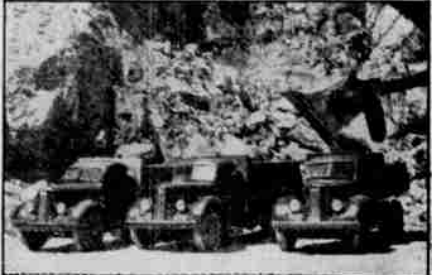
Half of the sea wall for the island was transported by GMC trucks from the quarry to sea-going barges that dumped the big boulders into place. Photos below show the trucks at work in the quarry and loading one of the huge barges.
