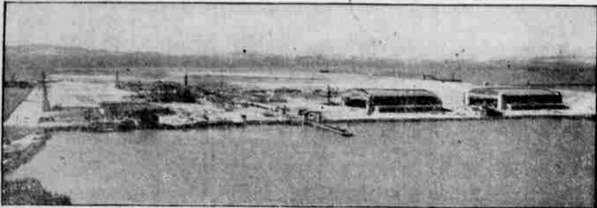
The 430 acre site of the Golden Gate International Exposition shown above is literally a magic island for it was made of material dredged up from the sea. After the exposition in 1939 it will be transformed into a fine municipal airport.
