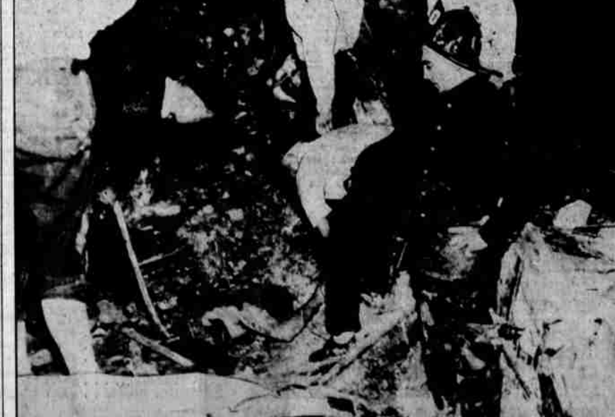
The collapse of two brick tenement buildings, on Staten Island, N. Y., brought death to 19 persons Thursday. Above, firemen are shown searching the ruins for bodies after the disaster, which investigators believe was caused by a plugged storm sewer under the buildings, causing the structures to be undermined by torrents of rainwater.
