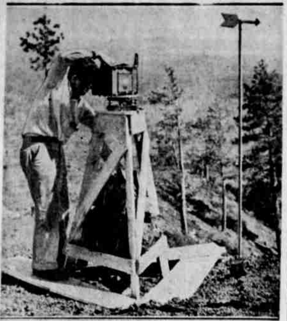
A special type of camera devised for photo survey work, is being used by the forest service in visual mapping, with oriented exposures being made from every lookout station in Oregon and Washington. The crew under Junior Forester Albert Ernst is making the photographic maps as an aid in speeding fire detection, location and arrival of fire fighters at the scene.
