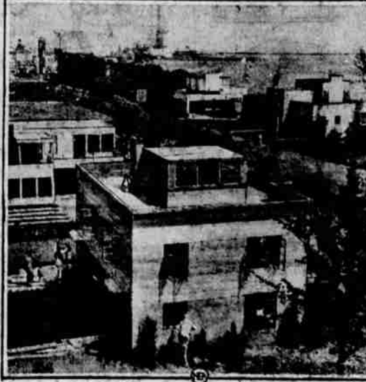
Four of eleven "tomorrow's houses" built of steel and other fabricated materials, that grace Chicago's Century of Progress are shown here, two on each side of the street. They are magnets for many visitors to the fair.
