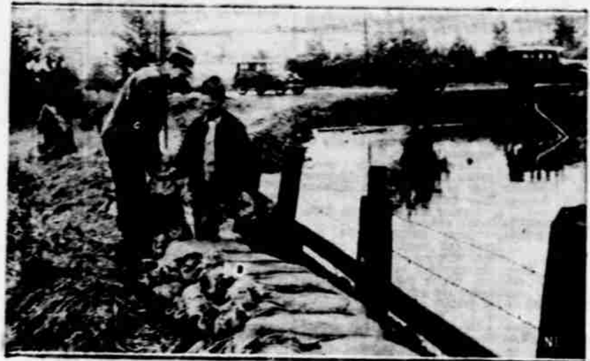
Heavy spring rains have swollen the Willamette and Columbia rivers and their tributaries until low-lying towns and farms have felt encroaching waters, and bridges have been lost. Photo shows farmers working to strengthen dikes along the Columbia near Vancouver, Wash.
