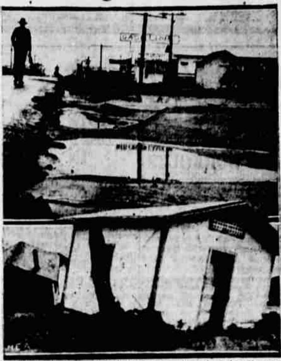
One known dead and several missing was the toll of this disastrous cloudburst which inundated Wellton, Ariz., recently. Rushing waters swept away a dozen cabins and tore out huge sections of the main street. Above, a view down Main street; below, tourist cabins left askew by the cloudburst.
