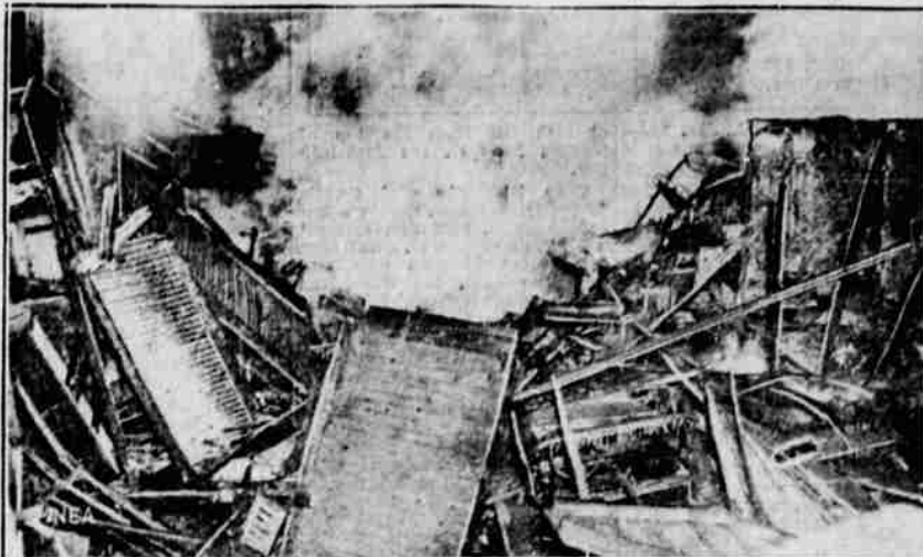
Four terrific gas explosions rocked the entire city of Monaca, Pa., near Pittsburgh, the other day, ripped a business block to bits and then started a fire which had the effect shown in this picture. Aside from the block that was destroyed, scores of houses were damaged, and 25 families were driven from the street. Damage is estimated at $225,000.
