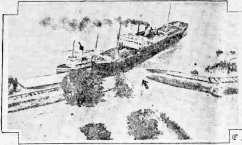
Swirling currents in the flooded Mississippi river caused the tanker "Inspector" to ram a levee at Union Plantation, Louisiana, forty miles below New Orleans, causing a torrent of water to flow through the break and driving 1,200 persons from their homes. Other levee cuts have been made deliberately near New Orleans to relieve pressure on the city's dikes. Arrow points to break made by steamship.
