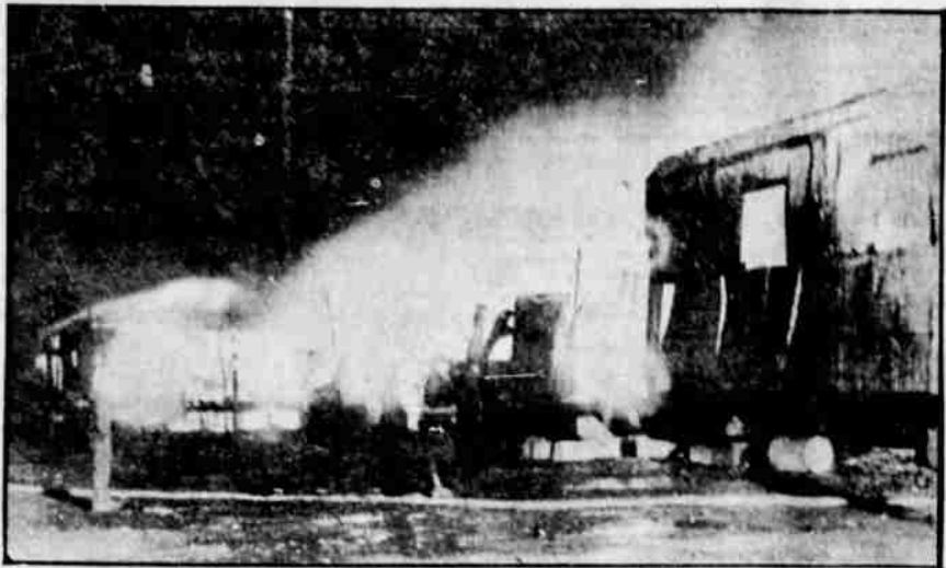
Picture of army cantonment barracks on fire at Governor's Island, New York, throwing lurid glare over harbor and lower Manhattan at dusk, causing Gothamites to believe a disastrous conflagration was in progress. Four structures were destroyed; eight men were injured. Telephotograph transmitted over A. T. & T. wires to Central Press and rushed by fastest service for publication.
