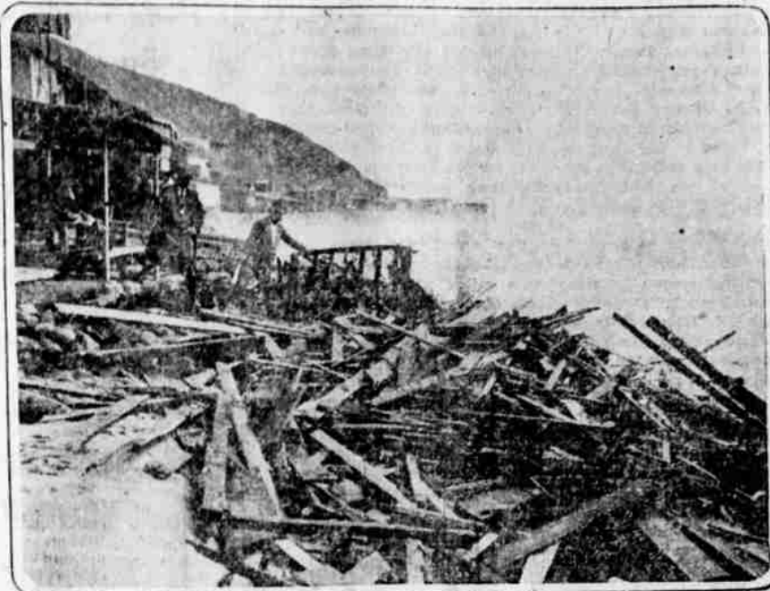
Damage amounting to thousands of dollars was caused by a recent storm that swept in from the Pacific Ocean, wrecking houses and damaging piers from Inceville to Palisades Del Rey, in the Santa Monica Bay district. Photo shows a part of the wreckage that was strewn along the shore for a distance of several miles.
