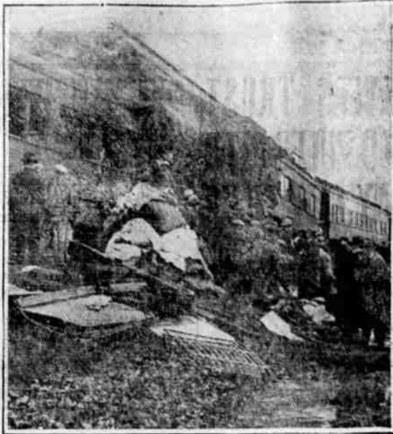
Engineer of the Merchantile Express is blamed for fatal collision of the train with a Washington-New York train on the Pennsylvania railroad at Monmouth Junction, N. J. He ran by a warning signal, investigators declare. Photo shows dead and injured being removed from telescoped sleeping cars.
