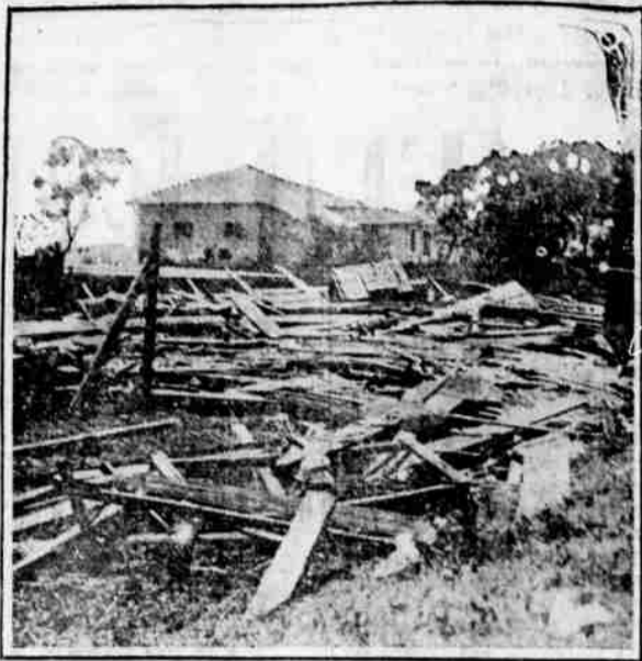
A section of Seabrook, on Galveston Bay, Texas, after a cyclone swept through the town, bringing death to several, and doing thousands of dollars worth of property damage.
