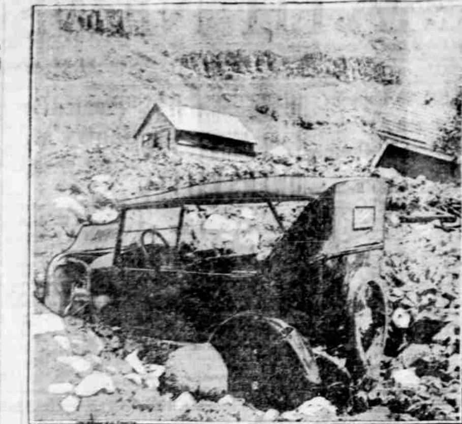
The force of an electrical, hail and rain storm turned Astin creek into a raging river, causing more than $250,000 damage to crops, buildings and stock in the vicinity of Lewiston, Idaho. Two children were washed from this auto and their bodies lost when a torrent poured over the hill, ripping away buildings but, strangely leaving them.
