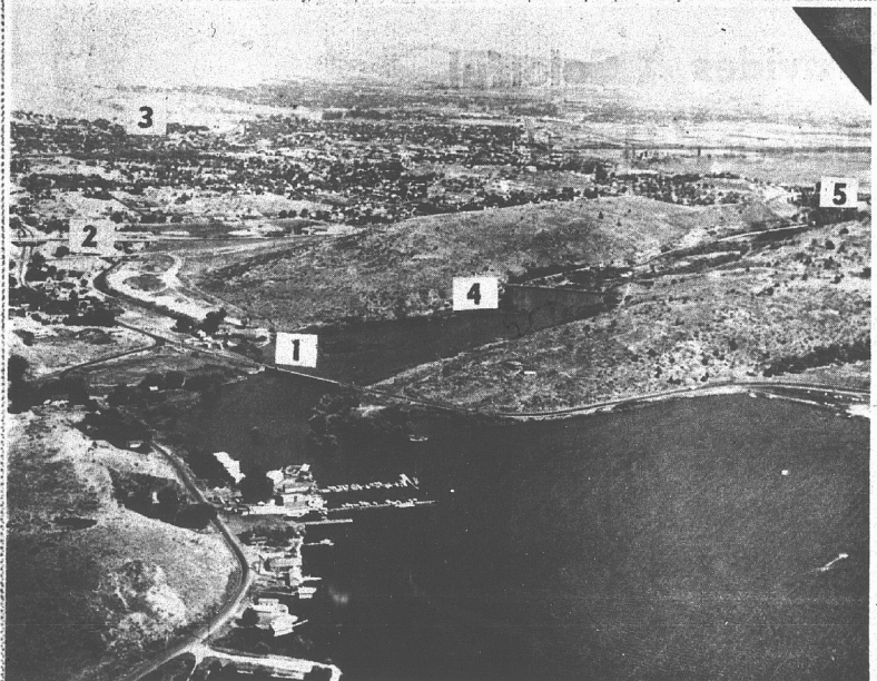
SOURCE OF WATER SUPPLY — This view of the southern end of Upper Klamath Lake shows the main facets of the irrigating process that provides water for much of the Klamath Basin agricultural area. (1) shows the intake canal which moves water from the beginning of Link River into the irrigation ditch. (2) is the location of the beginning of the long tunnel that carries about 7,000 feet to (3) where it emerges at Oregon Avenue and Eleventh Street. (4) shows the regulating dam on Link River and (5) is Lake Ewuna at the far end of Link River.
