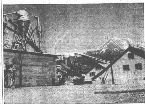
SPRAWLING INDUSTRY —The International Paper Company provides the town of Weed with a rather enviable economic base with an annual plywood and lumber production ranging in the millions of board feet and a $4.5 million annual payroll. Pictured above is one part of the Weed International Paper Company's plant.
