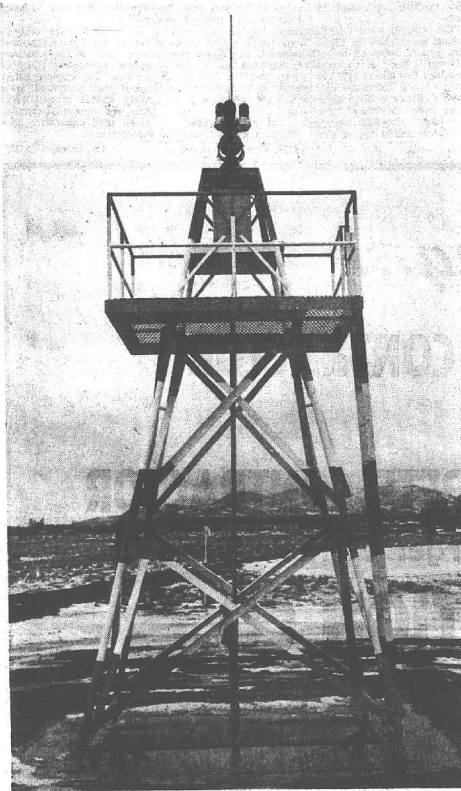
MEASURES VISIBILITY — The weather transmissometer is used to measure visibility for weather predictions made by Detachment Two of the 35th Weather Squadron at Kingsley Field. E. N. Alt constructed the two concrete bases and towers on which to mount the transmissometers. — AF Photo
