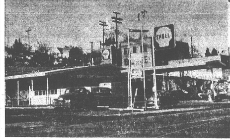
ONE OF TWO — This new Shell Oil Company station at 135 Main Street was one of two Shell operations completely reconstructed during 1964. This station is operated by R. G. "Whitney" Torgerson and maintained complete operation while the old building was torn down and the new one put up.
