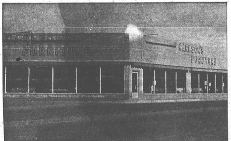
PLANT EXPANDED — Carlson's Furniture, 2405 South Sixth Street, completed remodeling its quarters in 1964, providing spacious new room for its retail furniture outlet and upholstery operation. The remodeling effort took place over a four-year period and completely revamped the firm's building. Latest addition provided 108 feet of window display space.
