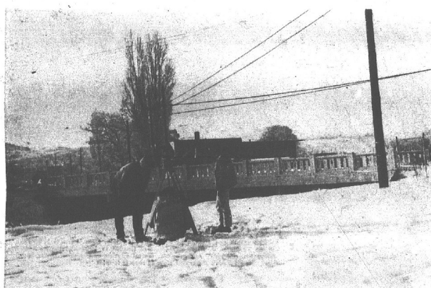
BRIDGE TO BE REBUILT — A state highway department survey party begins work preliminary to the replacement of the Main Street bridge in line with the construction of a new five-way intersection at Alameda Avenue and the
