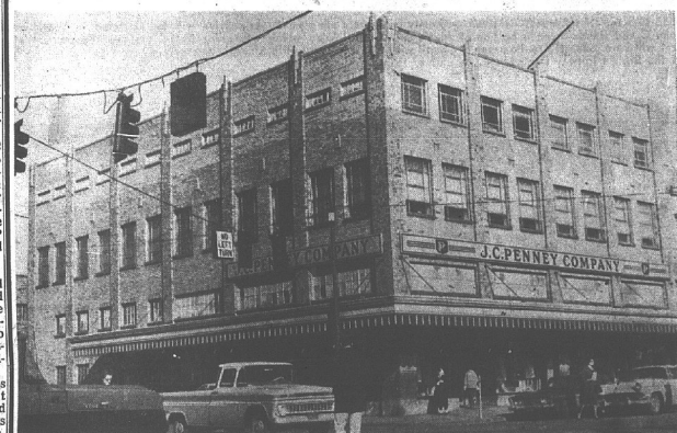
Located at 8th and Main, your Klamath Falls Penney Store is one of 1700 serving all 50 states. J. C. Penney Co. was founded in 1902 and the local store started here in 1937. A convenient, central location and elevator service to all floors, make Penney's the easiest place to shop in town!
