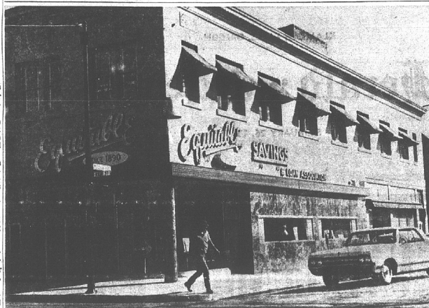
ENDS SUCCESSFUL YEAR — Equitable Savings and Loan ended 1964 on a high note and launched into its 75th Diamond Anniversary year in Oregon. This view shows the new quarters occupied by the Association during 1964 at the corner of Seventh and Main streets.
