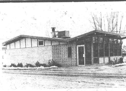
CALIFORNIA-OREGON TELEPHONE COMPANY BUILDING AT TULLAKE
