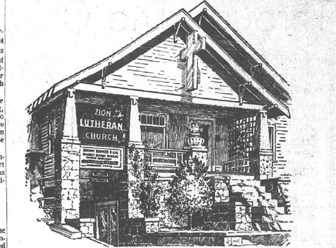
ZION LUTHERAN CHURCH Remodeled, now the parsonage.
