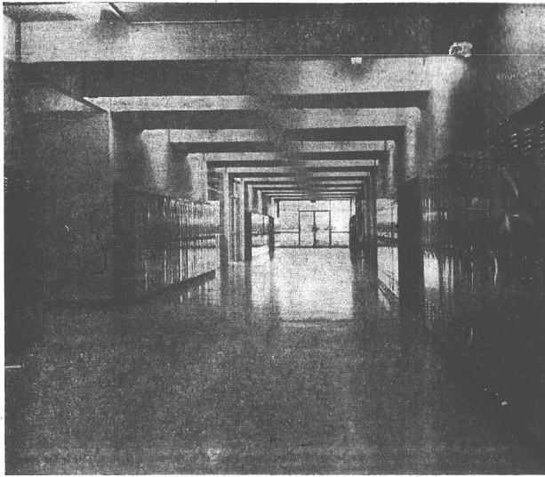
BROAD HALLWAYS — Broad hallways, giving ample room for foot traffic, are a feature of the new Henley Junior High School. The school was constructed at a cost of $418,072 by Cummings Construction of Grants Pass.
