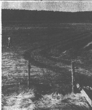
ROUTE OF CHANNEL — This view shows the route of the 3,000-foot-long bypass channel to be dug around a portion of the Klamath River in the vicinity of the Keno Regulating Dam. PPL has hired Morrison-Knudsen Construction Company to dig the channel, and expects it to be completed within 30 days. Flags show the survey route for the ditch. Les Carothers, surveyor, is shown in this photo. Duane Griffith is party chief of the surveying crew, which also includes Roy Allen.
