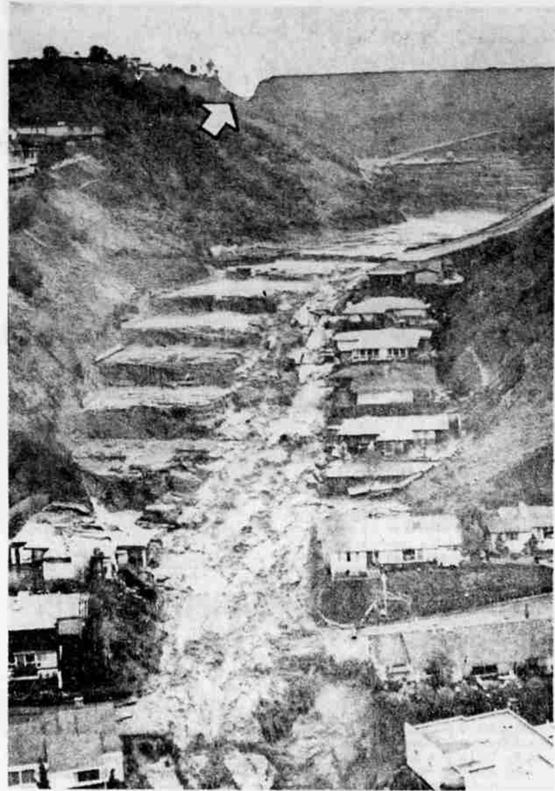
WATER RAVAGES AREA — On the right side of this street stand homes. On the left, all that is left is the pads where the homes were before the Baldwin Hills Reservoir Dam (background) burst, tossing houses and automobiles like toys onto the crest of the flood. The arrow points to the huge crack in the dam. At least 50 homes were destroyed by the gallons of water that roared through the broken fissure of the dam. Residents of the area returned today to sort through the debris. — UPI Telephoto
