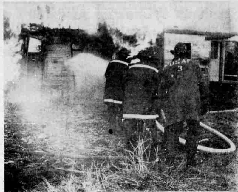
HOT SPOT — Four Kingsley Field firefighters edge up on a roaring inferno that once was a series of cabins on Market Street in Klamath Falls. The burning down of the old buildings gave firemen from the city department and the air base an opportunity to test their skills in extinguishing blazes. The firemen did their job well and often had to turn off their hoses to keep from putting out the fire before the buildings were leveled.
