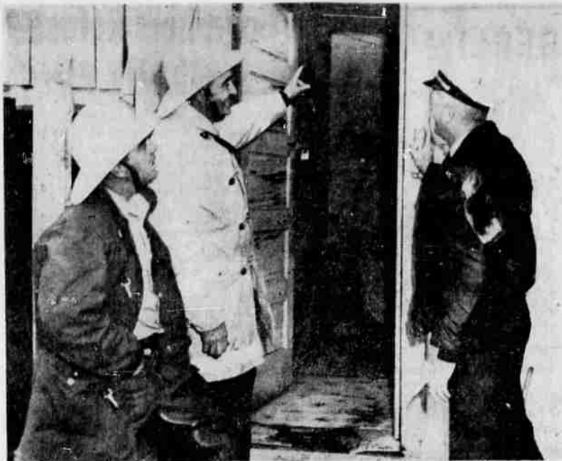
NEW ROLE — Officers and men of the Klamath Falls and Kingsley Field fire departments normally are concerned with the job of putting out fires. But Saturday it was their task to set fires as they destroyed a series of condemned buildings, using the structures for training purposes during the fire. Shown here are (left to right) Capt. John Mathews and Chief Geno Gheller of the city department and Chief Howard Larman from Kingsley as they inspect one of the cabins shortly before the torch was put to it.
