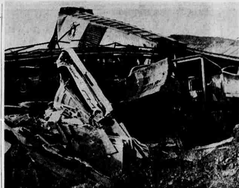
DESTRUCTION BEGETS DESTRUCTION — Bulldozers were used Monday afternoon to clear the Great Northern-Southern Pacific track 10 miles north of Klamath Falls of wreckage from Monday morning's train wreck. Traffic was resumed on the line Monday evening, 15 hours after the wreck of more than 30 cars. Here, a dozer pushes away the remains of a 1964 automobile and some sheet gypsum. The car was one of 15 riding on a wrecked flatcar.
