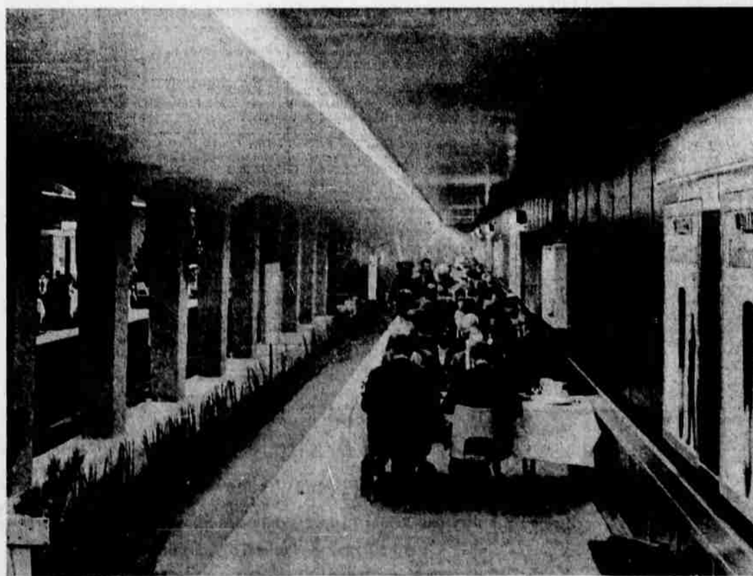
SUBWAY SUPPER —The still-unfinished Leuvehaven subway station in Rotterdam, Holland, offers a novel setting for a dinner for persons working on the tracks. As soon as the tracks are laid, the walls will reverberate with the sound of rushing trains, hardly the spot to sup. They'll have to enjoy the sweet repose as long as it lasts.
