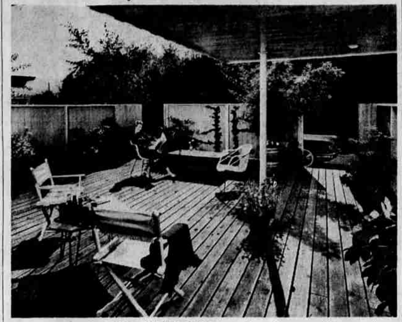
DECK MAKES CHARMING ENTRANCE YARD — The right approach to your home might be a wood deck like this, which levels grade between street and front door. Handsome entrance deck of weathered 2x6 Douglas fir boards is also a perfect lounge spot. Tall privacy windscreens are tongue-and-groove cedar siding in 2x4 frame. Home owner: H. C. Nachand, Portland. Architect: Burton J. Goodrich, AIA, Portland.
