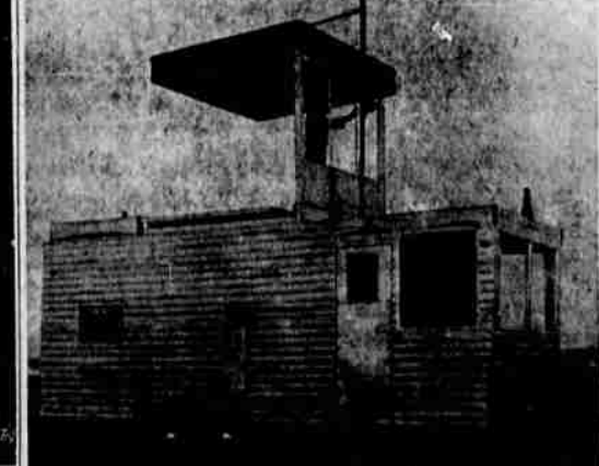
FIRE TRAILER — Portable lookout station features tower which can be raised in 15 minutes.
