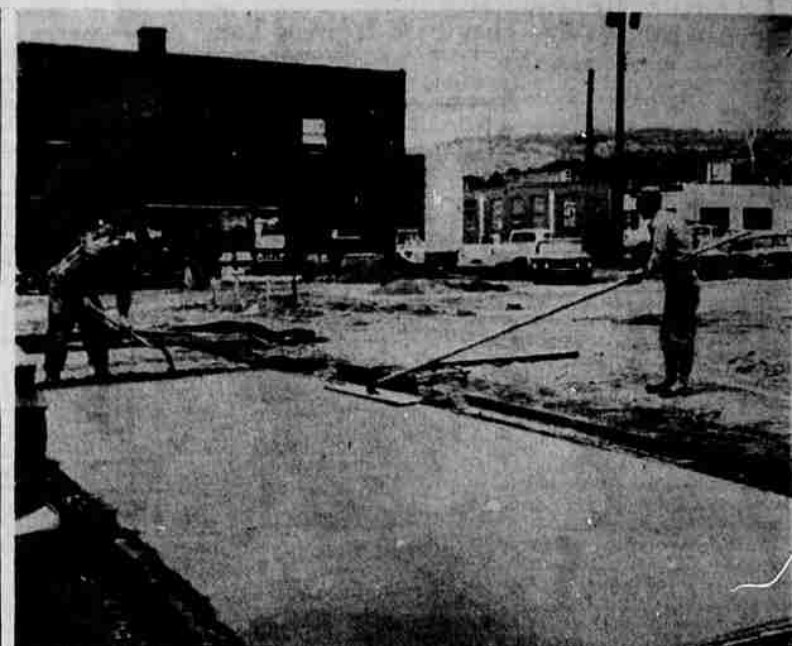
NEW MACHINE SHOP RISES — A cement slab was being poured at this site on South Sixth Street when the photographer happened by a short time ago. The building being constructed will house an automotive machine shop of Moty and Van Dyke, Inc., and, according to Kasper Moty will be the "most modern, best equipped shop in this territory." The building will cover over 3,700 square feet, and is being independently contracted. The building will be constructed by Bennington Steel Company and will be masonry and steel. Moty indicated that the machine shop adjacent to the main structure on Klamath Avenue is inadequate and the new building will house this operation. The building is scheduled for completion in early October.
