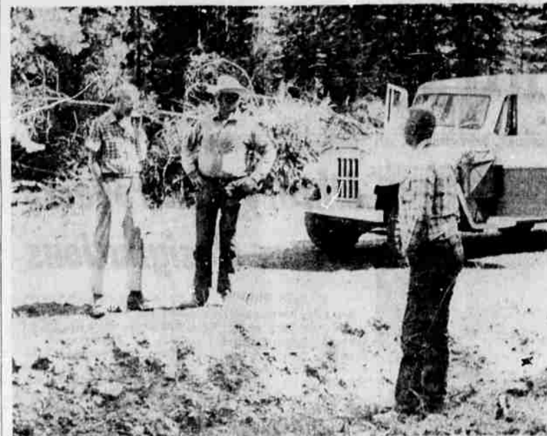
WATER PROGRAM — Viewing the Weyerhaeuser Company's water development program, begun as an integral part of access road construction into virgin territory at upper Long Creek near Silver Lake, are Fred Goeller of Weyerhaeuser and Buck and George Carlson, Summer Lake ranchers. Water from these developed springs and seeps is used for fire-fighting, recreational facilities, and livestock. The Carlsons were part of a group on a recent trip arranged by the Fort Rock-Silver Lake Soil Conservation District.
