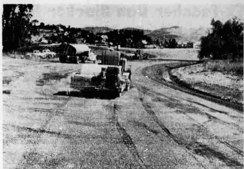
partner in the home with Richard Dilling. Far right, a view of the Riverside Street approach to the new west side bypass being constructed by the Lillebo Construction Company at an approximate cost of $861,000.
