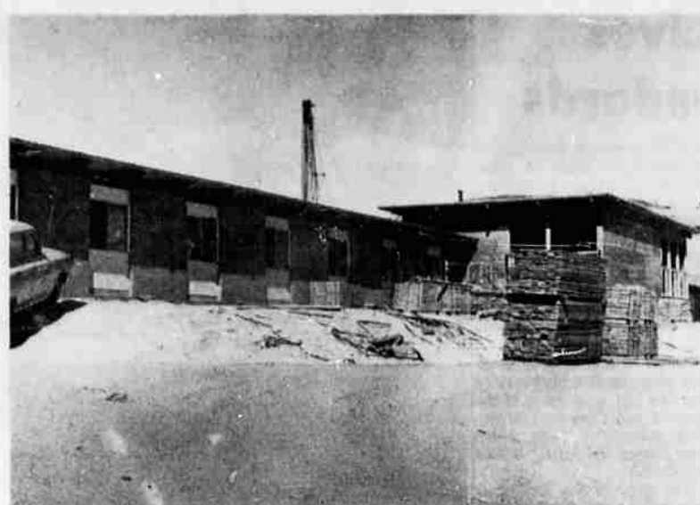
Center view is the new nursing home being built adjacent to Main Street near Ponderosa School at a cost of $300,000. It is being constructed by the Brostherhouse Construction Company with Virgil Cumbo, Wenatchee, Wash., general contractor and
