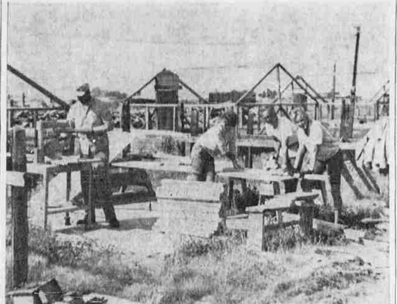
BUILDERS AT WORK — Constructing new tent frames for the Malin Migrant Center wasn't so difficult after the materials were measured, cut, and assembled in "pre-fab packages." The project was undertaken by youths in the Presbytery of Southwest Oregon as a six-day pioneer work camp experience. Working on the assembly-line, from left, are Rev. Ethan Whitman, counselor, Malin; Erin Lorton, Medford; Rev. Laing Sibbet, dean, Klamath Falls, and Dru An Graff, Medford. All of the lumber and nails were donated by Klamath Basin concerns.
