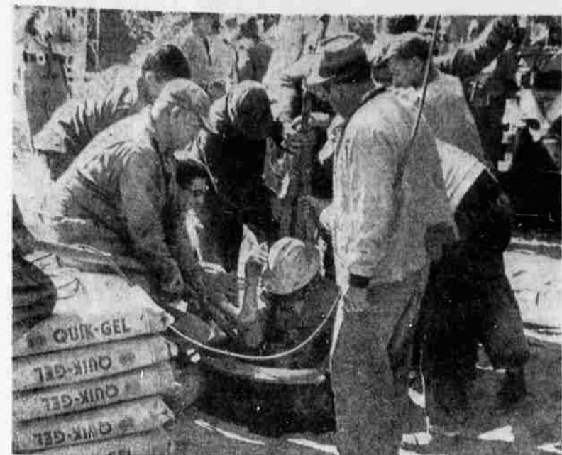
INSPECTION JOURNEY — Rescue worker John Adams is brought up from the holed-out hole that was drilled toward miners David Fellin and Henry Throne, trapped more than 300 feet below the surface. Adams was lowered in a special harness 37 feet into the hole to inspect the drilling which is widening the hole so the miners can be hauled out.
