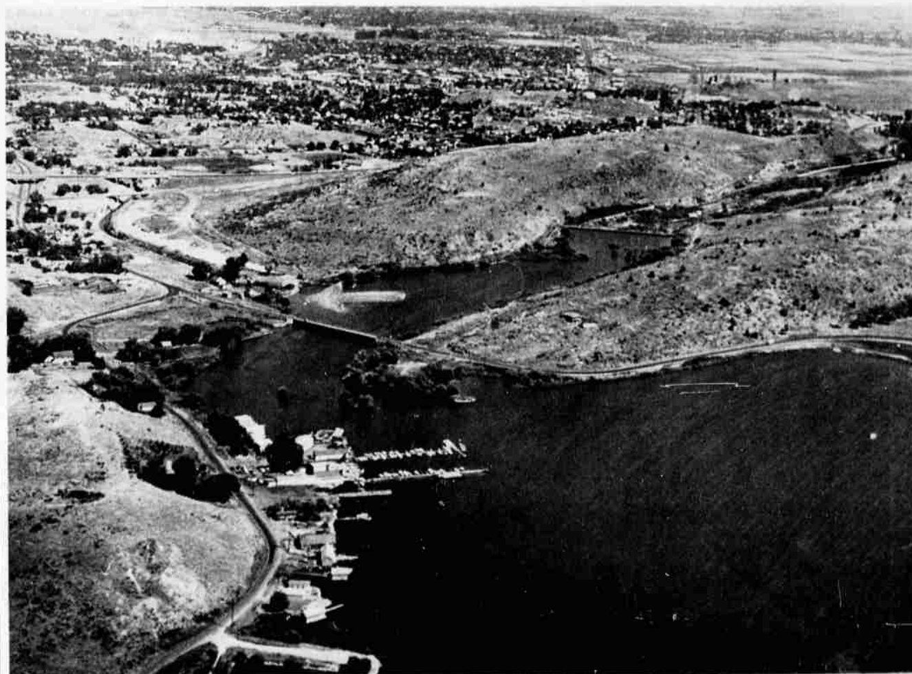
WHERE IT ALL COMES FROM — Arrow points to the intake where water is drawn from the southern end of Upper Klamath Lake into "A" canal and thence into the whole system of canals that distributes water throughout the Klamath Basin. Currently, about 300,000-acre feet of water is drawn out of the lake annually for the Klamath Irrigation District.
