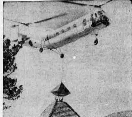
WHERE'S THE STEEPLE? —How to place a 650-pound steeple atop the meeting house of Carmel Valley Manor, Calif., is shown by this helicopter. The entire project cost $4.5 million. It is a retirement community.
