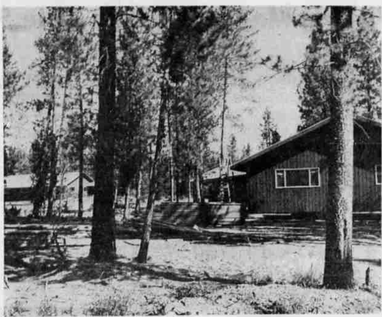
CHILOQUIN DISTRICT WORK NEARS END — The new headquarters of the Chiloquin Ranger District in the Winema National Forest were nearing completion today as employees of the Quality Builders Company, Klamath Falls, were in the final stages of work on the office building, warehouse, a 10-man barracks, oil house and four dwellings. The contract deadline is Sept. 27. Another contract for an equipment storage building and three dwellings was completed July 25 by the Kyia Construction Company of Portland. Part of the $200,000 building project which started last March was financed from Federal Accelerated Public Works Program funds.
