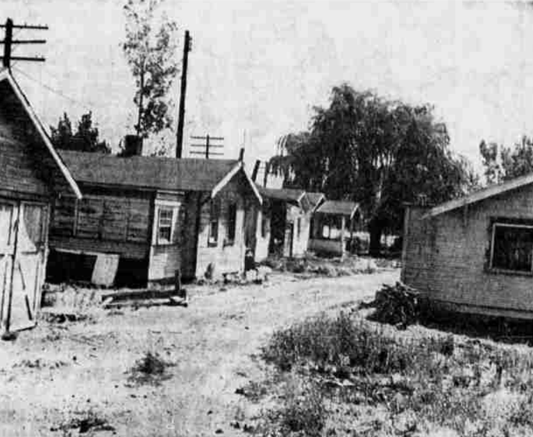
CONDEMNED — Four of these Portland Street cabins owned by Frank R. Weaver were ordered condemned by the city council last week as part of a continuing campaign to rid the city of substandard structures. They are typical of the buildings that have been destroyed through city action within the last year and a half.
