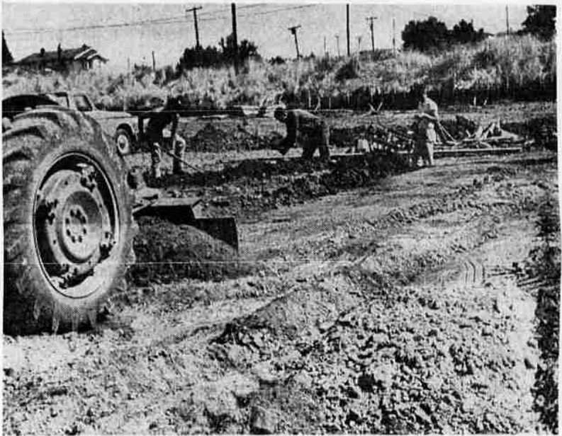
PLAYLOT WORK UNDERWAY — The Parks and Recreation Department is developing its play lot at the corner of North Second and McKinley streets and work crews Thursday began building the sidewalk encircled sand-pit that will be over 30 feet in diameter. The first phase of the automatic irrigation system was installed and the system should be completed next week. Grass will be planted by the end of the month. Several pieces of play apparatus will be placed in the playlot after it is turfed and landscaped, Gary Woodring, park director, said.
