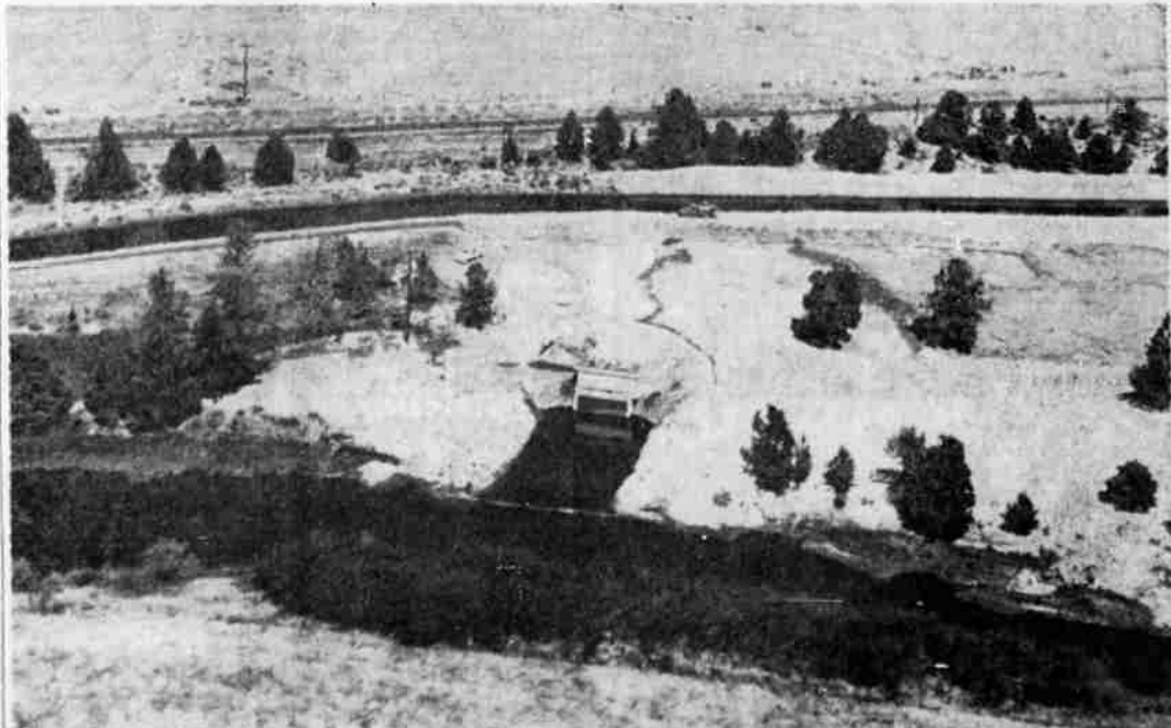
DEDICATION SET — This is the new Stukel Pumping Plant, 12 miles southeast of Klamath Falls, where dedication ceremonies for the Klamath Project Extension were planned this afternoon. Main speaker was to be Floyd E. Dominy, commissioner of the U.S. Bureau of Reclamation
