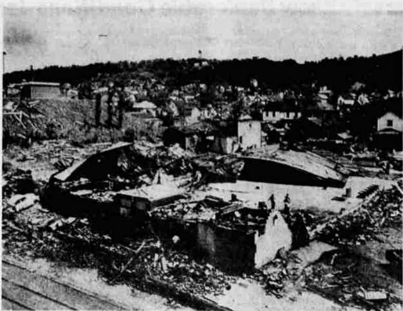
75 INJURED AT RINK — Workmen clear the debris from what remains of the Glassport Roller Rink which collapsed late Saturday when it was hit by tornado-like winds of 89 miles an hour which ripped through the suburban Pittsburgh town. Police say that 75 persons were injured when the roof fell in.
