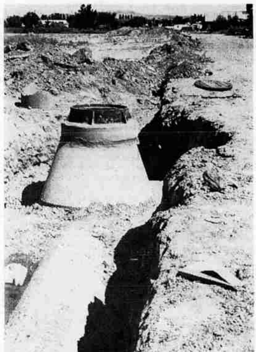
PREPARING TO CATCH RUNOFF — Storm sewers are being constructed on Washburn Way, Pershing Way, Avalon and Austin streets to catch rain water runoff in these areas that previously were without the facilities. Sanitary sewer projects are also planned for the Mountain View section. The Mountain View work will cost approximately $25,000 and the contract was awarded to the W. D. Miller Construction Company.
