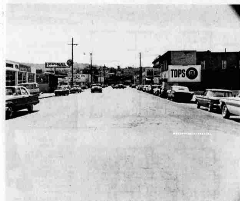
MAIN STREET BEFORE AND AFTER — These two shots show Main Street before, left, and after, right, the new slurry seal surfacing that cost the city approximately $950. Slurry seal projects completed in the last few weeks included South Fourth, Fifth and Sixth streets.
