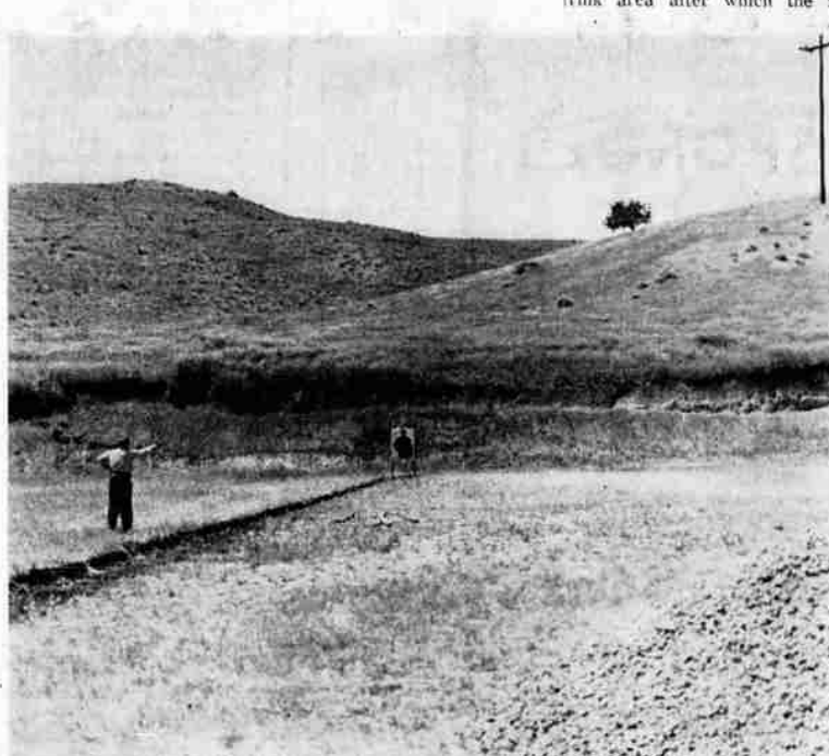
POLICEMEN BUILD RANGE — City policemen worked almost two years during off-duty hours constructing this outdoor shooting range off the OTI road. All the bulldozing and grading was done by policemen with borrowed machinery. The target holders were constructed and the targets put in place recently. Five runways, like the one at the right, will be asphalted in the near future. Planting grass and digging a well are planned after the runways are paved.
