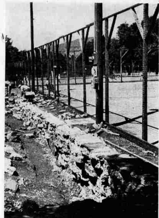
PARKING AREA RETAINING WALL — A crew from the City Recreation Department is working on a retaining wall at the parking lot next to the newly resurfaced Moore Park tennis courts. The resurface work cost an estimated $500, but the wall is being constructed mostly with city owned material.
