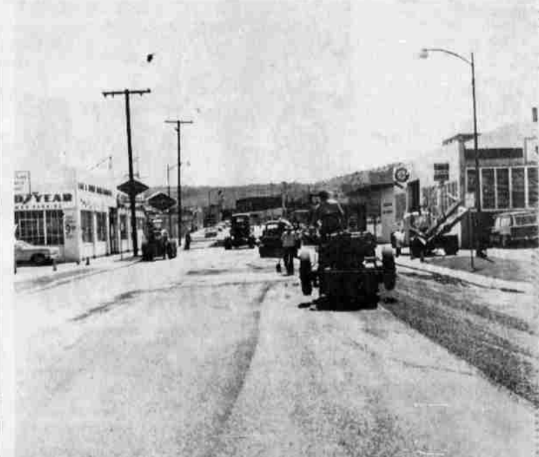
KLAMATH AVENUE IN TOP SHAPE — When the City Street Department started prying into Klamath Avenue they found out how not to build a street. On the original project, necessary base rock wasn't used as a foundation and the street failed in many places. Where it failed it was replaced with sufficient base rock and the rest was resurfaced. The project cost an estimated $4,500.
