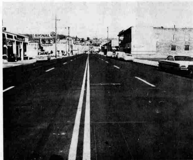
Forthcoming paving projects will include Laguna Street, Worden Street, Van Ness, Tiffany, Benson, Euclid, Birch, Avalon and Calhoun streets. Asphalt paving is planned for most of these streets. The slurry sealer is a makeshift piece of equipment designed and built by City
