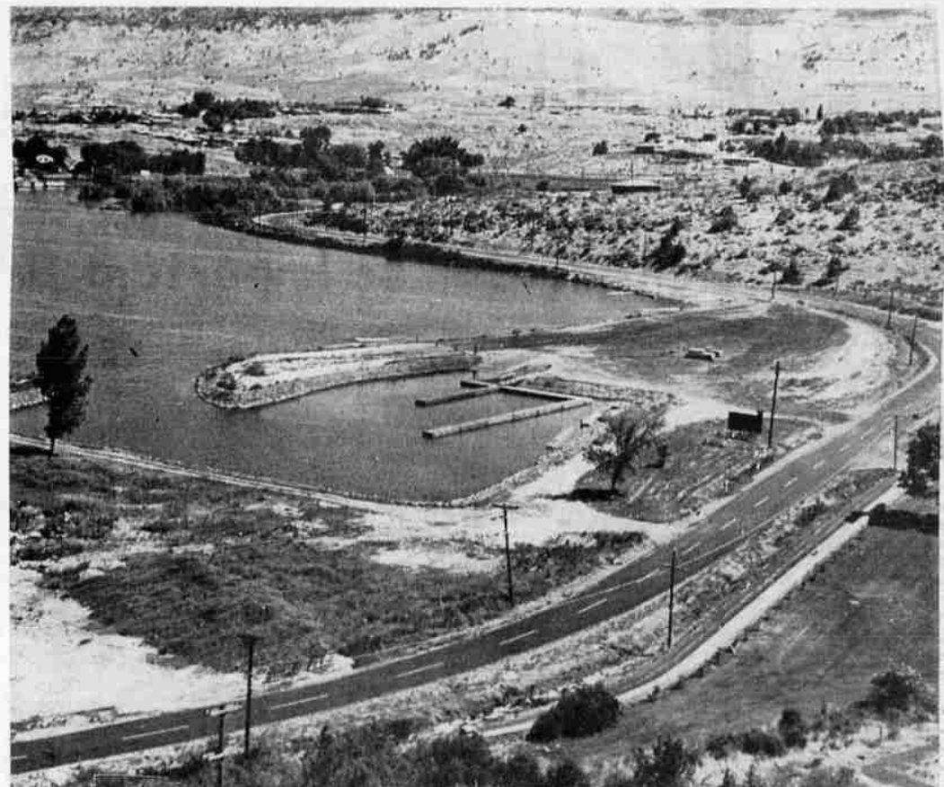
NEW DOCKS JUT INTO MARINA — New docks supported with styrofoam flotation were launched at the Moore Park Marina this month giving boaters plenty of room to secure their lines while loading and unloading passengers. The docks provide almost 250 feet of docking space for boats of all sizes. The Klamath County Parks Commission provided $2,700 of the funds, taken
