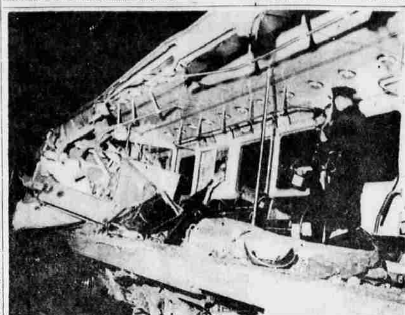
TRAIN WRECKED — A policeman looks over the wrecked interior of a passenger car following train collision at Harrison, N.J., early Wednesday. Two persons were killed and 31 hurt when the commuter train rammed a switch engine at a crossing. The train had 42 passengers and a crew of four aboard. — UPI Telephoto
